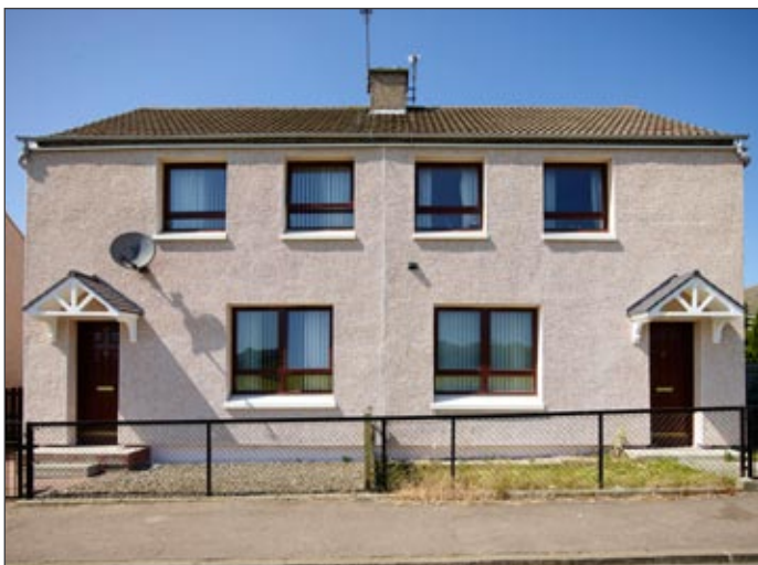
Social Housing Refurbishment Project: Heavy Duty NSC3 EWI System with Dash Aggregate finish
